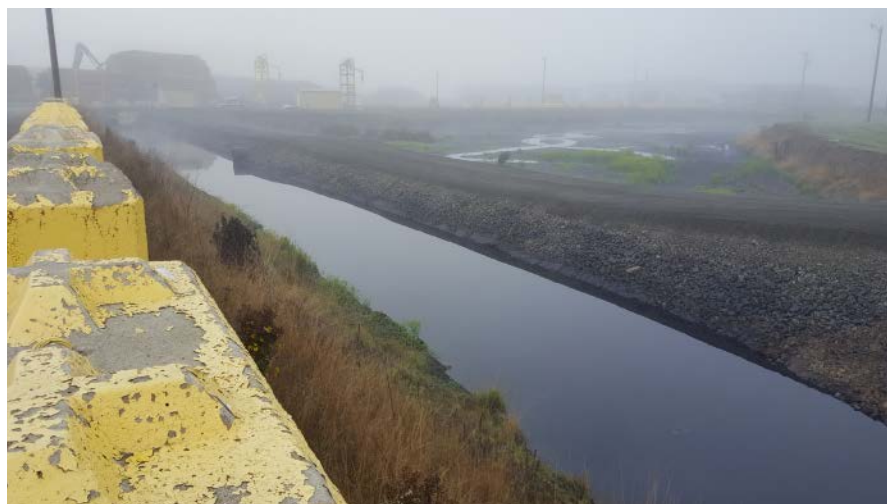
Image of the Seneca Saw Mill detention pond with permeable block edge and sediment drop.
