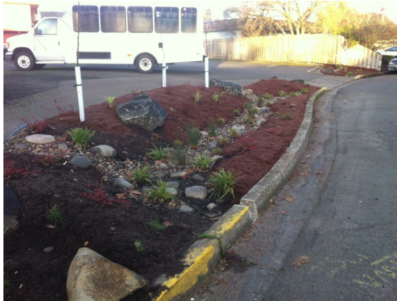
This stormwater swale replaces excess asphalt to slow and treat runoff pollution from a parking lot before it gets to Amazon Creek.
