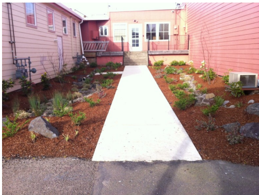
Turf area converted to swales to treat stormwater before heading to Amazon Creek
