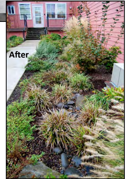
Turf at Davis Properties converted to beautiful swales to treat stormwater
