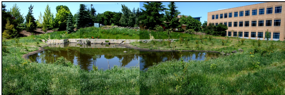
Thermo Fisher Scientific removed a 3 story building with plans to fill it in with lawn. Thanks to employees who went through BRING's Re-Think program who reached out to LTWC, we created a swale, retention pond and upland meadow that supports wildlife and cleans an acre of stormwater before it flows into Amazon Creek.
