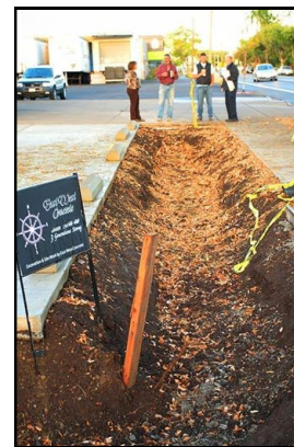
Joe's Garage is installing a rain garden that will manage all of the stormwater from their new parking and garage.
