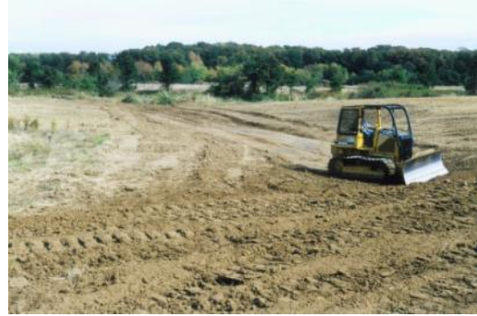
Bulldozer removes fill disconnecting historic Coyote Cr.
