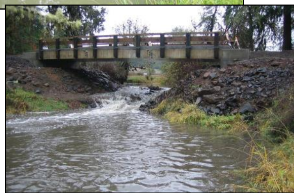
Before & After: The top photo shows the two foot drop at the culvert's outlet in the summer. Now the crossing is passable to fish year round .
