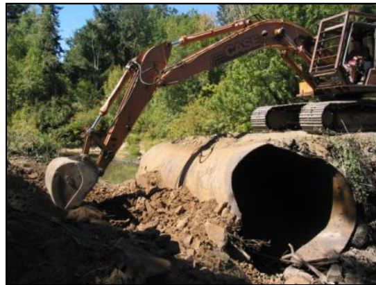
An excavator removes the undersized culvert that blocked fish passage to 46 miles of upstream habitat.
