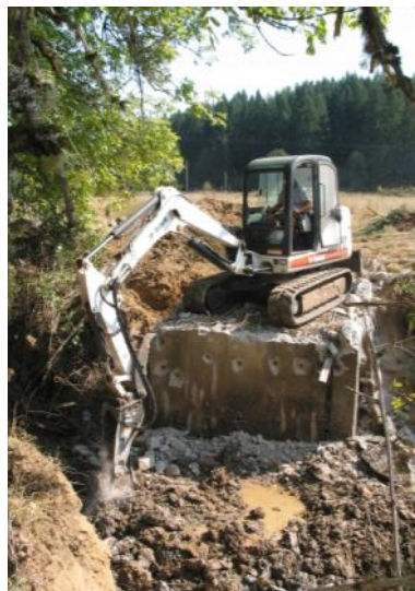
To left: concrete dam being broken up for removal; To right: Bridge slabs being placed by a crane.
