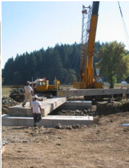
To left: concrete dam being broken up for removal; To right: Bridge slabs being placed by a crane.
