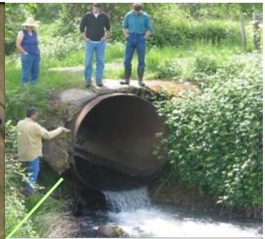
Pre-project: This undersized, perched culvert blocked fish passage to 5 miles of cutthroat trout habitat.
