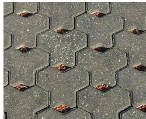
Permeable Pavers provide an alternative hardscape that infiltrates stormwater — EcoFriend.com
